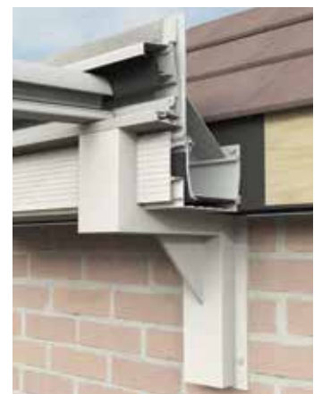
Custom designed gallows brackets are sometimes required
