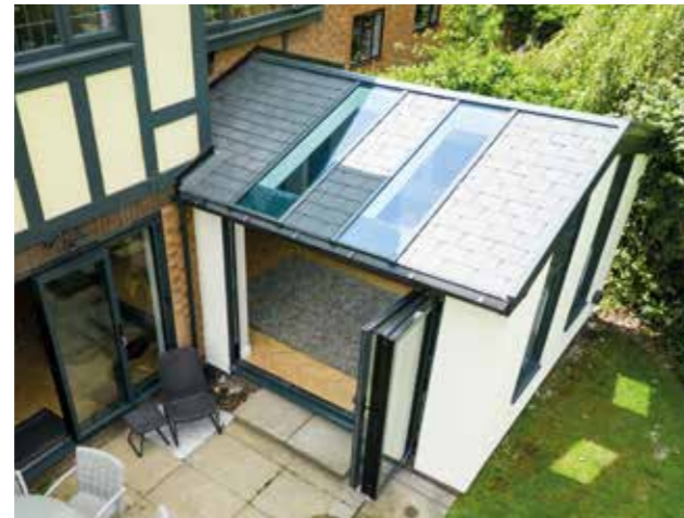
Tiled Roof | P22
